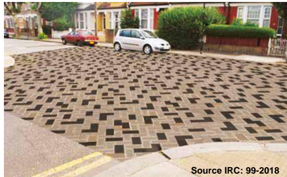
Figure 10 Textured Paving over Raised Crossings
